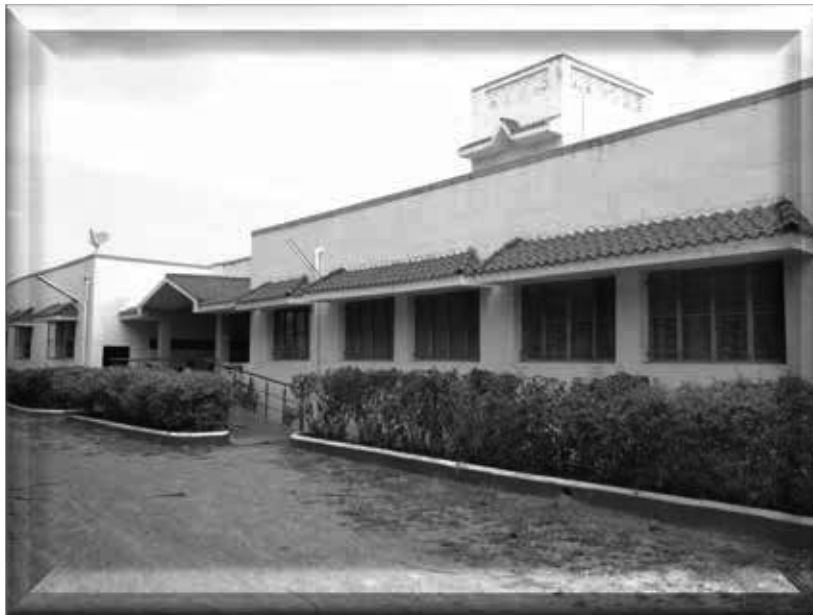
SABIN-PATHWAY REHABILITATION BLOCK AGILI, CHENGALPET DT. INDIA
