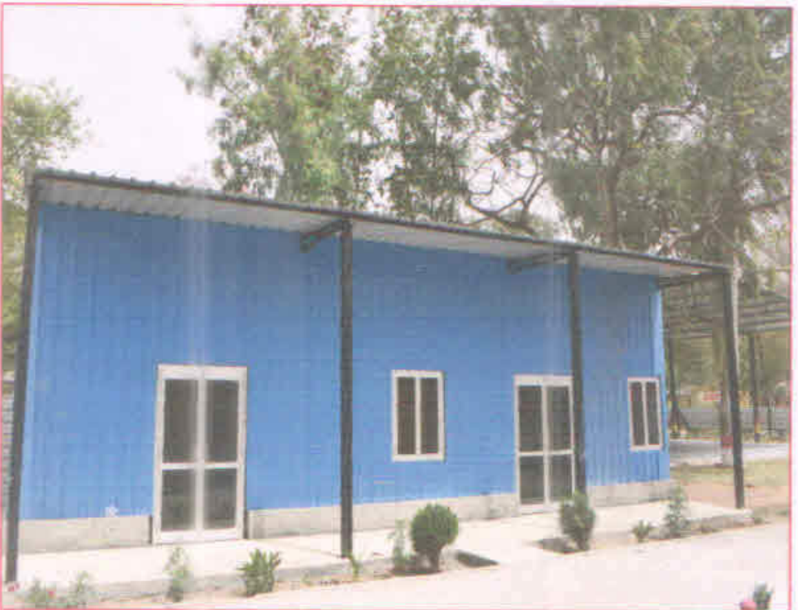
FABRICATED SHELTER WITH WARANDAH
